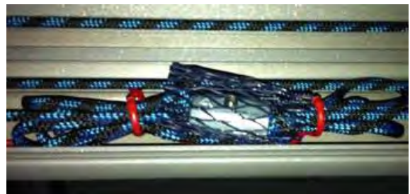
Tensioning rope fixed with cable ties
