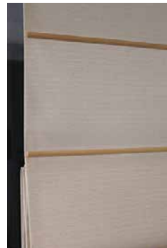
Timber Battens Front
